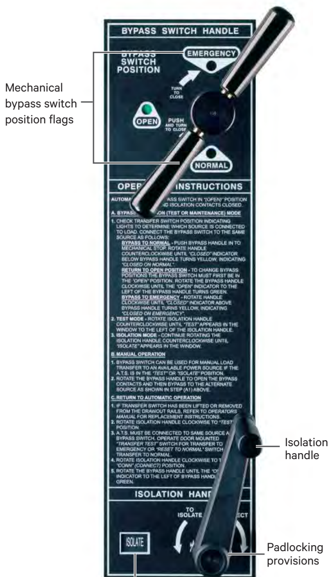
Mechanical isolation handle position window (connected/test/isolate)
